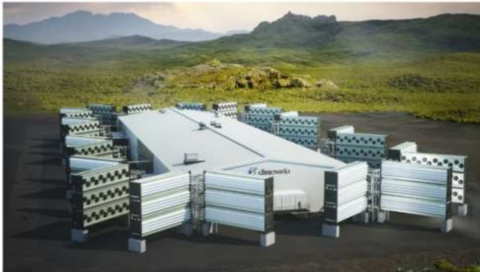
Figure 13: Illustrative rendering of 36kt S-DAC plant by Climeworks, named Mammoth, currently under construction and to start operation in early 2024.
